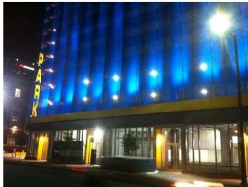
*ACTUAL PICTURE OF PARKING GARAGE*
