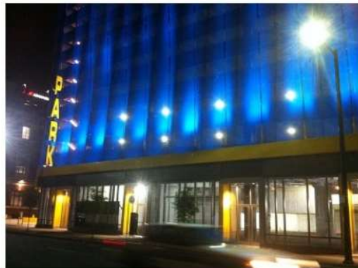
*ACTUAL PICTURE OF PARKING GARAGE*
